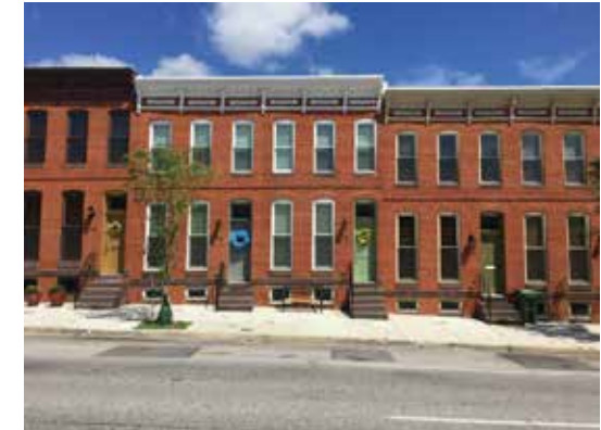
RESTORE SURROUNDING NEIGHBORHOOD
