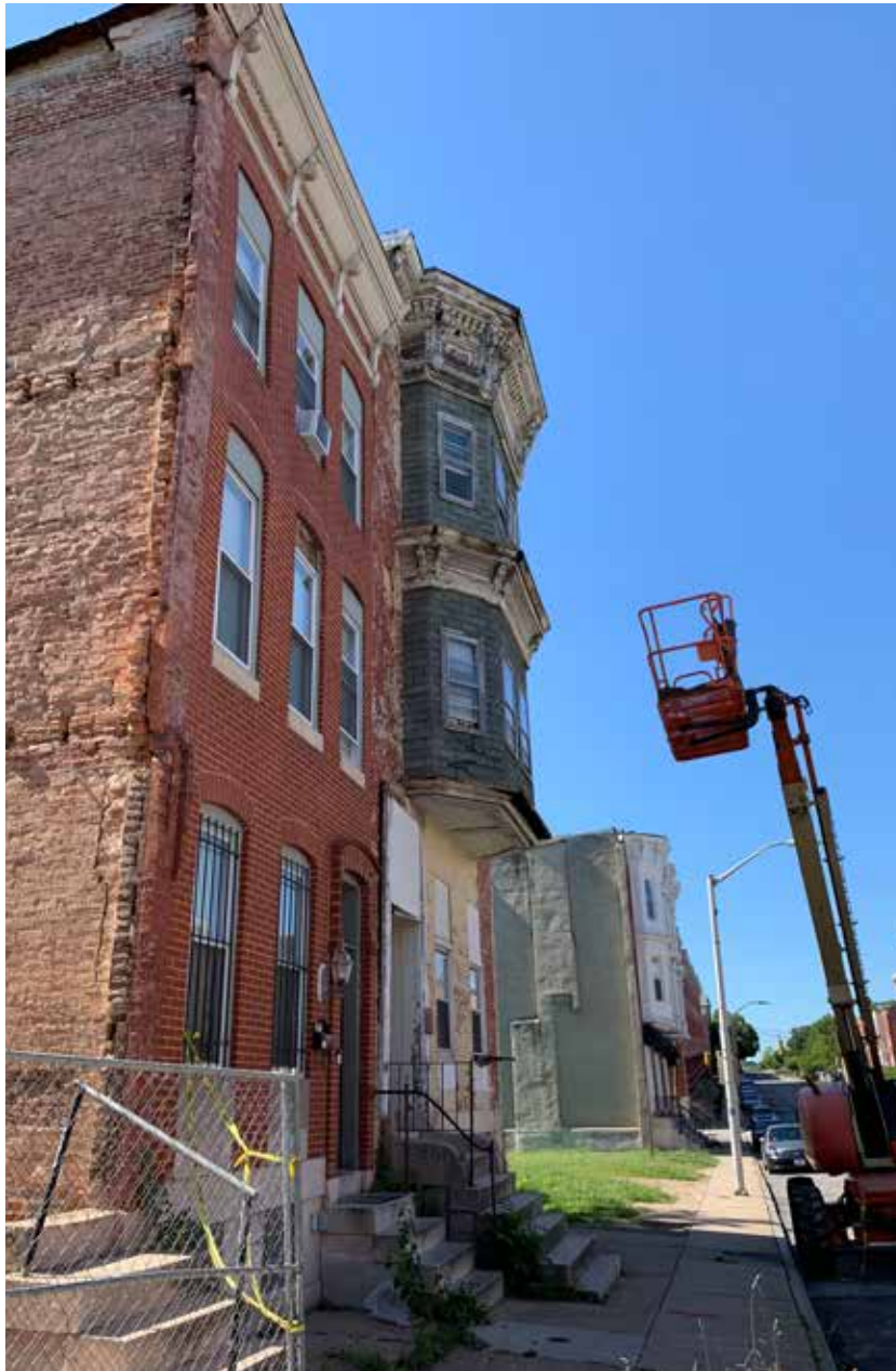
Home restoration and infill along Fulton Ave.
